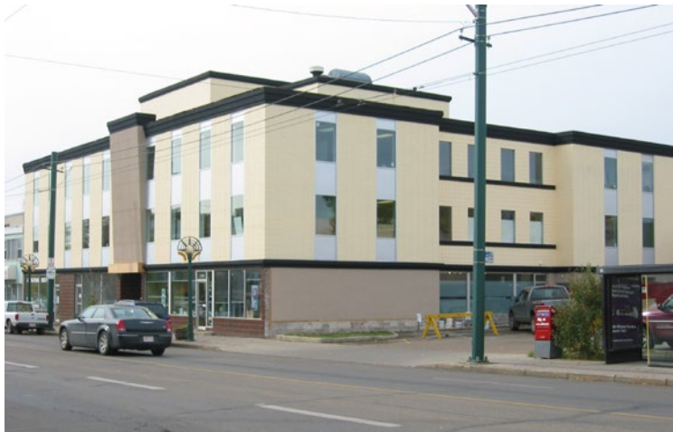
The Zurich Building Re-Face, downtown Edmonton.
